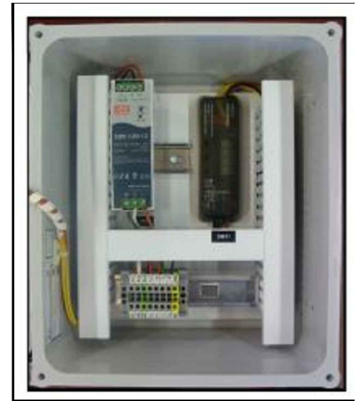
TYPICAL INTERIOR VIEW
